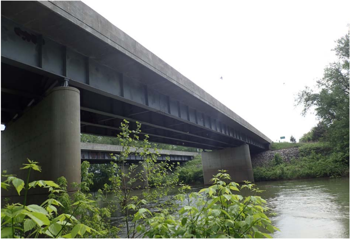
Typical view of span 2.
