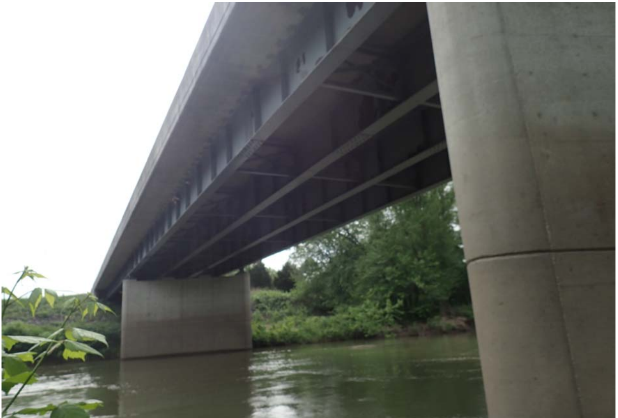
Typical view of span 2 and pier 2.
