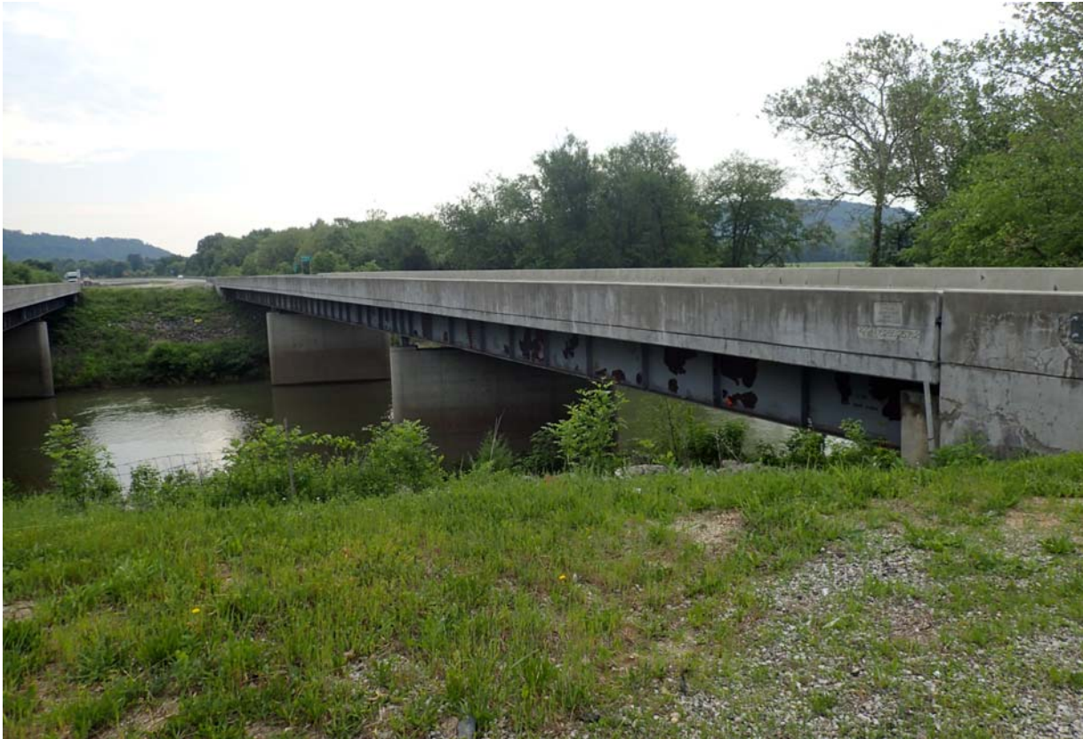
View from the downstream end of abutment 1.
