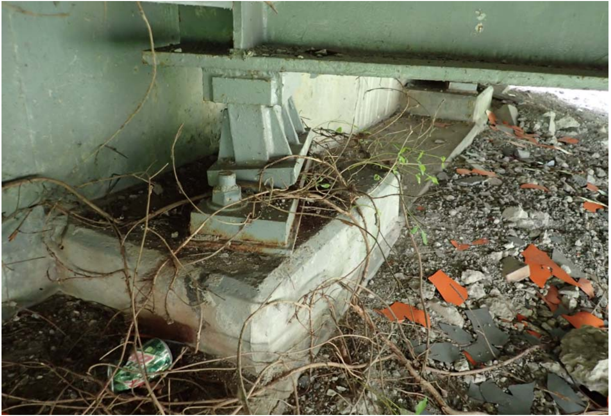
Typical view of bearing 3 from upstream at abutment 4.
