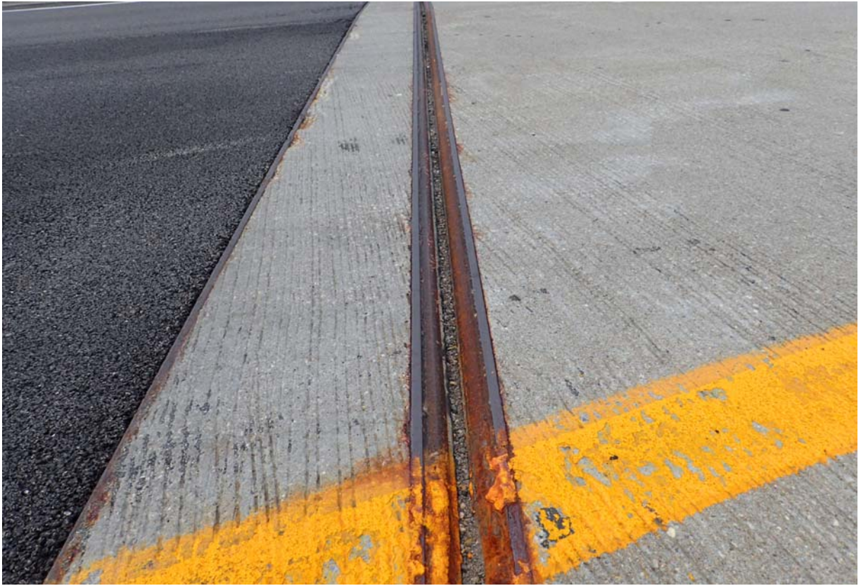
View of the transverse joint at abutment 4.
