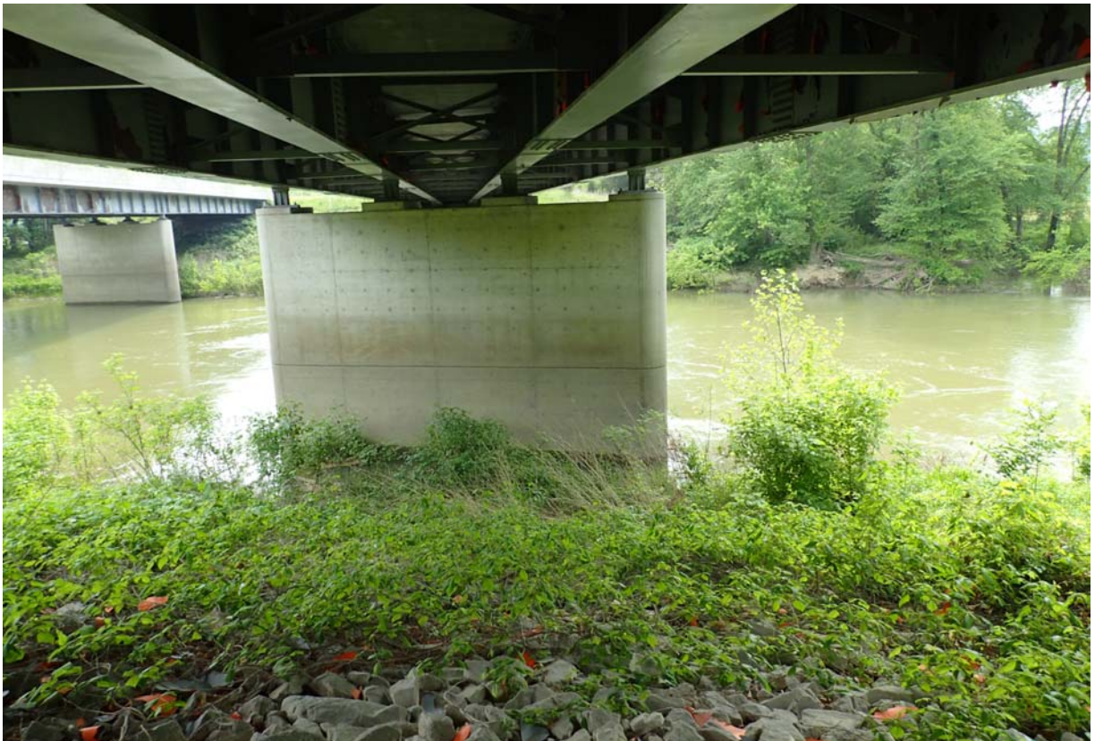
Typical view of pier 2.
